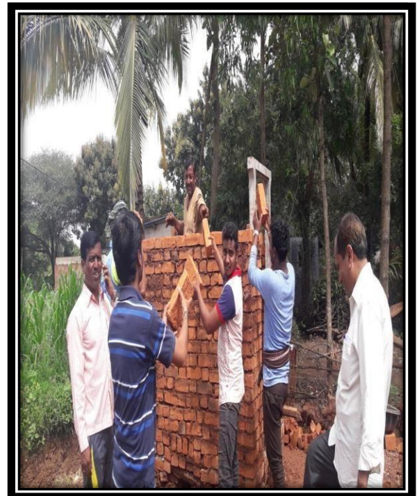
NSS Volunteers Constructing Toilets at Mangalagatti Village
